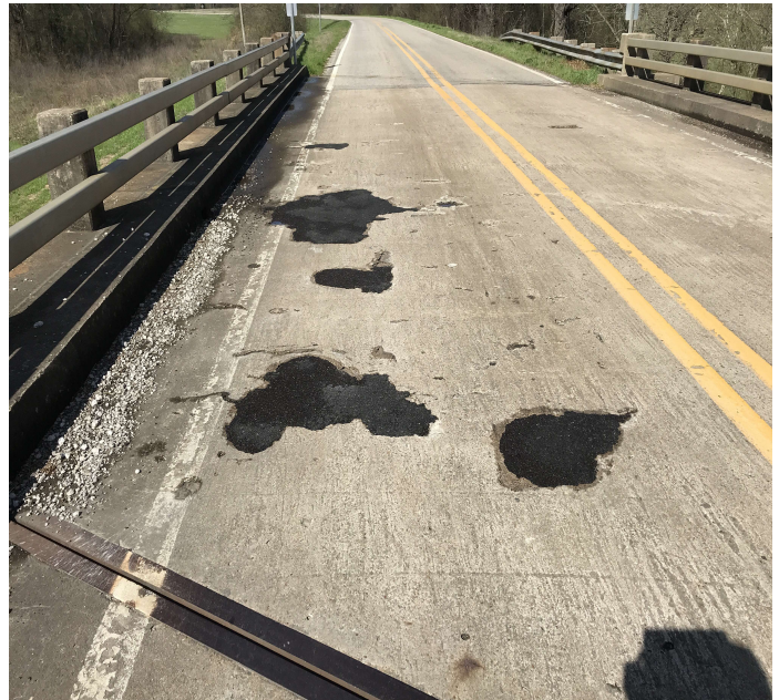
PHOTO 6 Description Span # 1 Rt temporary asphalt patches.
