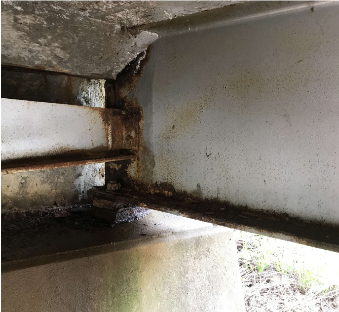
PHOTO 3 Description Bent # 5 Beam # 5 layers of flaking rust.
