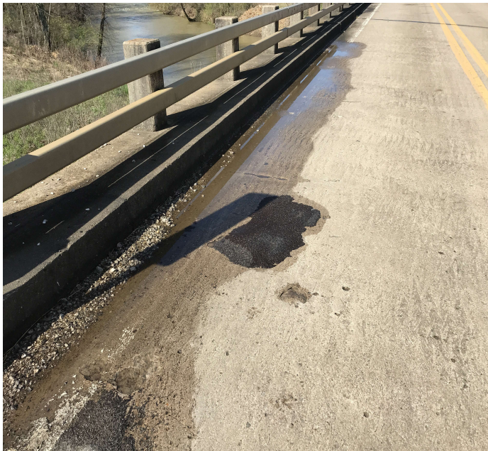
PHOTO 1 Description Span # 4 Rt spalling, delamination and temporary asphalt patches.
