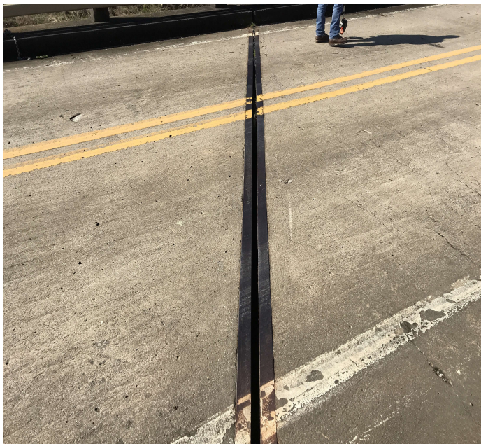
PHOTO 1 Description Bent # 4 joint seal failure.
