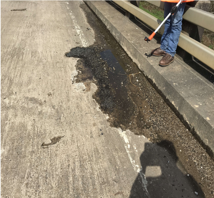
PHOTO 7 Description Span # 1 Lt spalling in the gutter.
