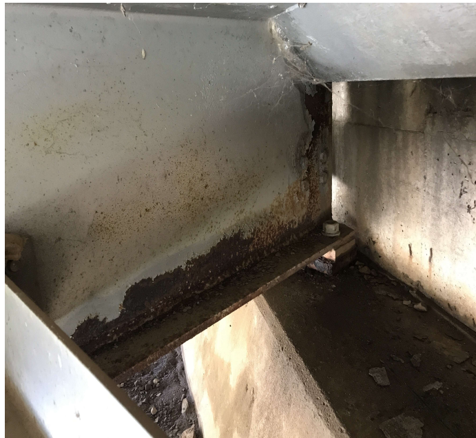
PHOTO 1 Description Active corrosion at the Beam ends typical.
