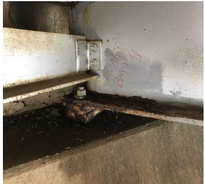
PHOTO 2 Description Bent # 5 Beam # 4 active corrosion with layers of flaking rust.
