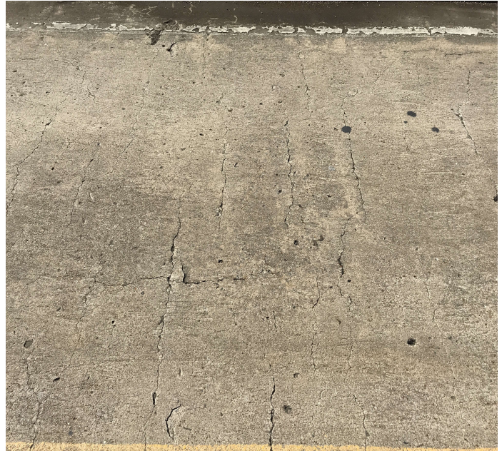
PHOTO 5 Description Sealable deck cracking.
