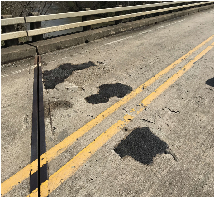
PHOTO 4 Description Span # 2 adjacent to Bent # 2 spalling with exposed reinforcing steel and numerous deteriorating repairs.
