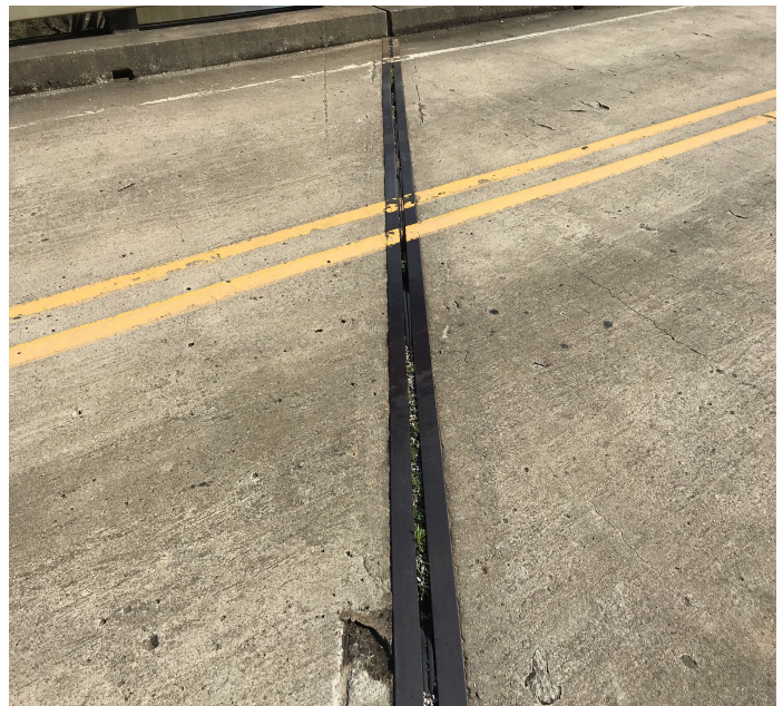
PHOTO 2 Description Bent # 3 joint seal deterioration.
