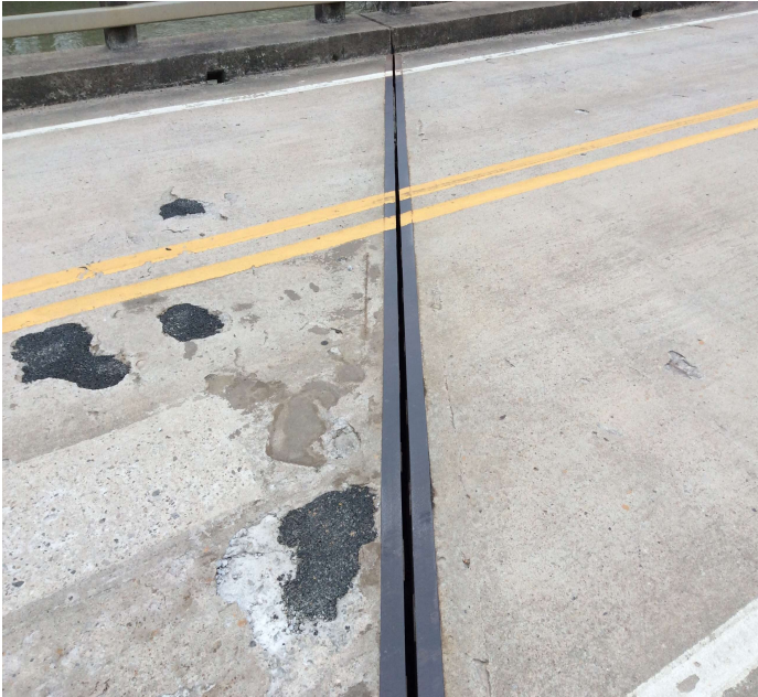
PHOTO 3 Description Bent 2 deck joint seal missing
