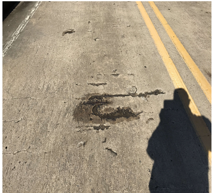
PHOTO 2 Description Span # 3 Rt spalling with exposed reinforcing steel.
